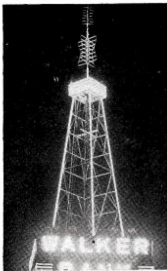
KDYL's super turnstile or "bat wing" antenna. Tower is outlined with red neon tubing.
